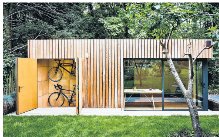
This garden office (from £21,595), designed by Green Studios, is clad in cedar boards, has a sedum roof and incorporates a bike shed
