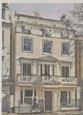
A new-build house with a piano nobile in Notting Hill, west London, is on sale for £25 million through Rokstone
